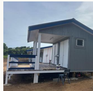
Figure 10. New Wash Facility
