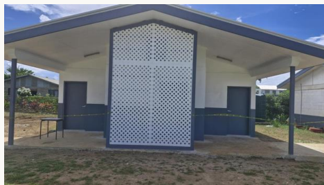
Figure 2. New Wash facility
