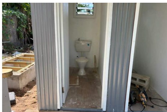
Figure 14. New Wash Facility
